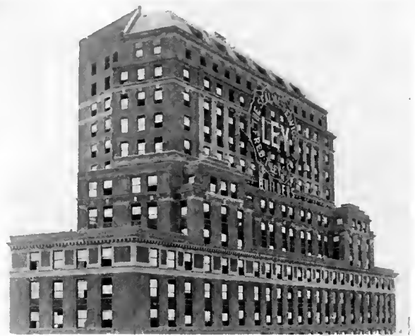
FIG. 5. UPPER STORIES OF FISK BUILDING
